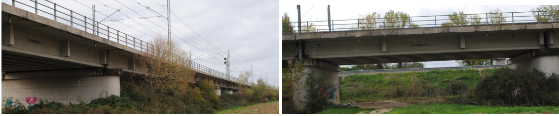
Fig. 3. Views of the viaduct and of a sample span.
