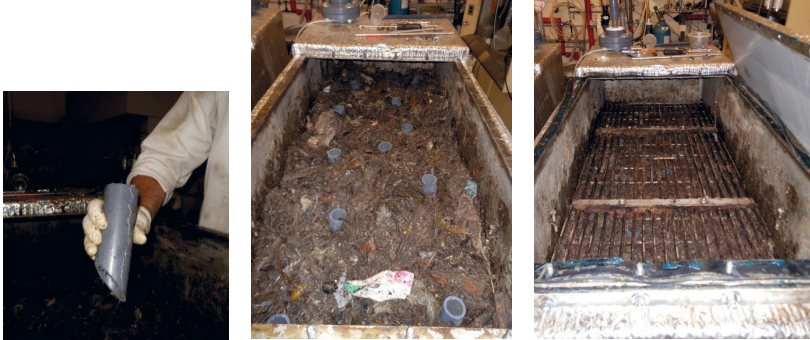
Figure 8.7-7: Pipe segment drainage channels placed and installed beneath the grating (Source: InnoTech)
