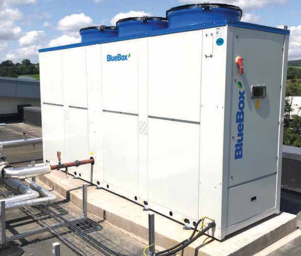
Left: An example showing the ZETA REV HP XT used in the Enniskillen PCC project in Co Donegal.
