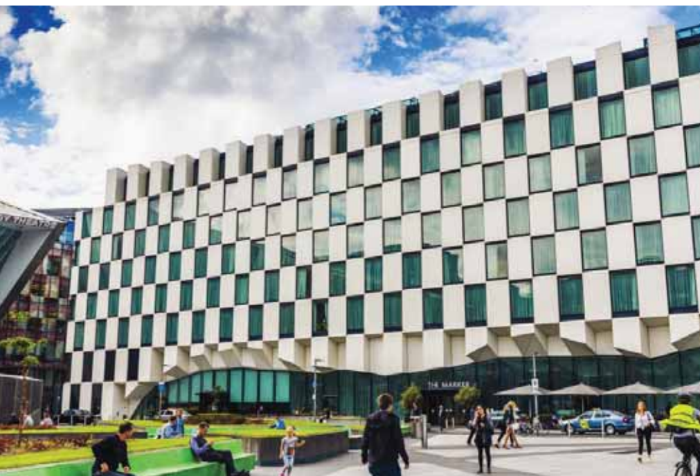
Lightsolutions carried out medial on-site emergency lighting works and certification at the Marker Hotel, Dublin.
