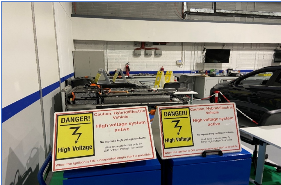
Figure 27 Hyundai Ireland, electric vehicle technical training centre. Lithium-ion batteries, electric vehicles, diagnostic tooling and equipment, create significant costs for educating actors in this new technology (MMcGuinness, 2021).
