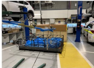
Battery lifting crane
