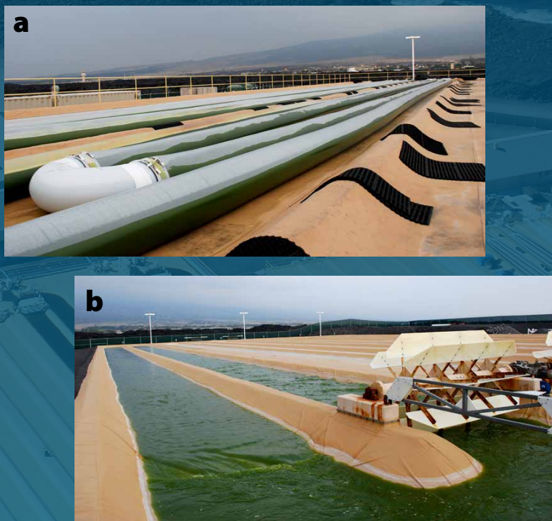
FIGURE B1. The Cellana Kona Demonstration Facility (KDF) where demonstration-scale cultivation experiments using ALDUO™ technology were conducted. (a) Closed-loop photobioreactors. (b) Open raceway ponds.
