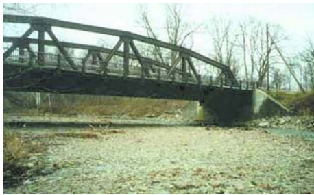
Fig. 2. Bentley Creek Bridge (2000).
