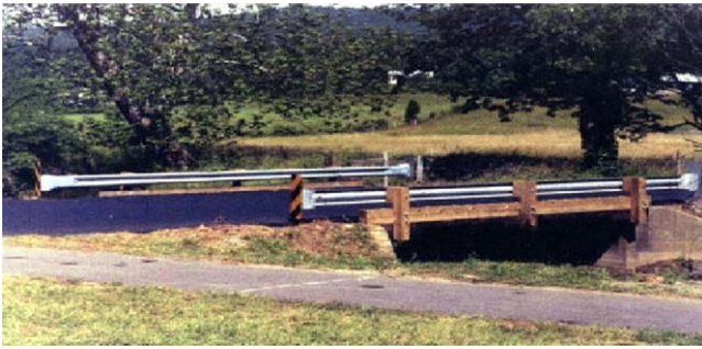
Fig. 1. Tom's Creek Bridge (1996).
