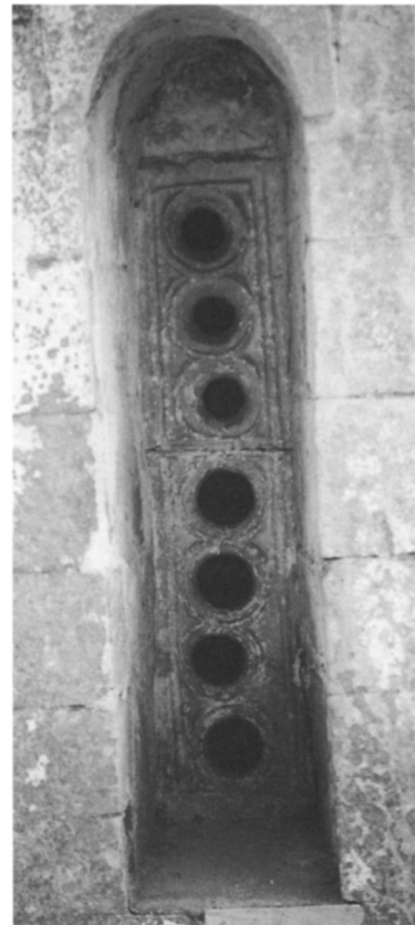
Fig. 10 Apsidal window with stone transenna. San Pietro ad Oratorium , Capestrano, 12th century (photo by author)
