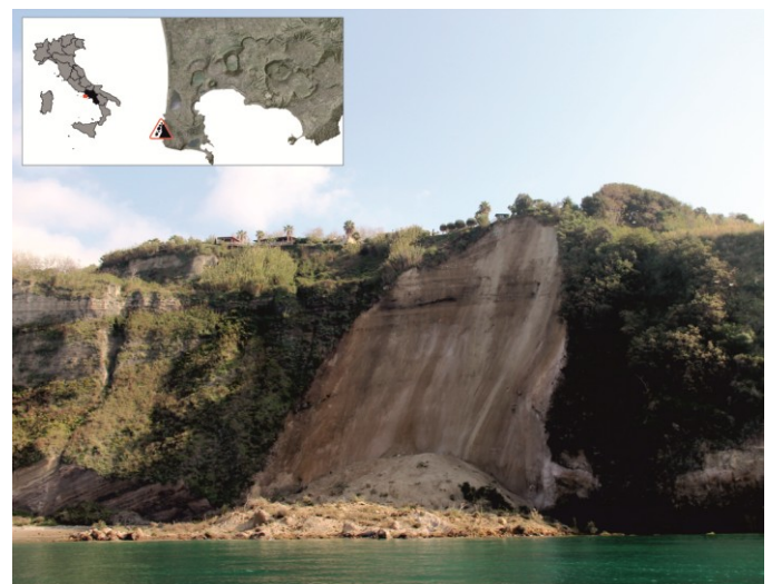
Fig. 1 - Photo of the landslide taken from a boat; inset map shows the location of the study area.
