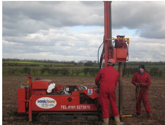
Figure 7: The Sonic-bore drilling rig at work at the Shelford site
