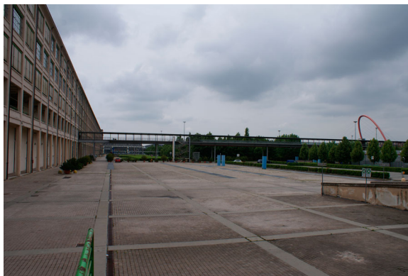
Figure 8. Lingotto, the pedestrian bridge and the Olympic arch. Source: photo by the authors, 2016.
