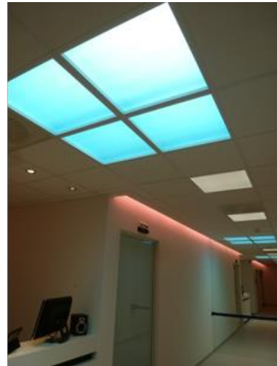
Fig. 1: Virtual skylight in a hospital corridor
