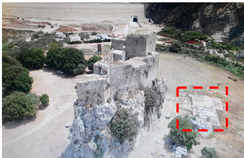
Figure 2. Mseilha Fort showing the mill to the right of the castle in red.
