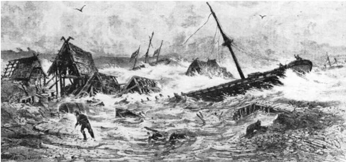
Figure 1: The damage caused in Haffkrug located at Lübeck Bay/German Baltic Sea Coast during the storm surge of November 1872 (Illustration: C. Rettich und C. Heyn).
