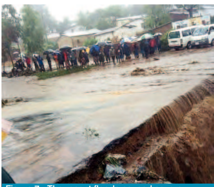
Figure 7 - The recent floods caused severe damage to important infrastructure in Malawi
