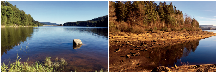
Figure 2. Schwarzenbach Reservoir at maximum operation level (left) and during water level lowering (right)
