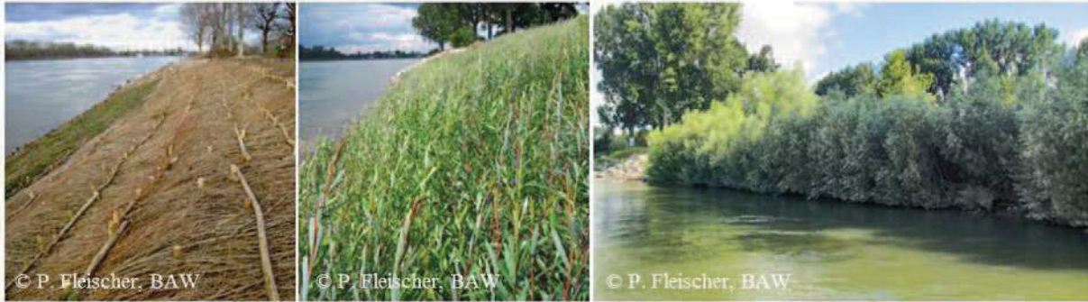
Fig.1: Willow brush mattresses 2011 after installation (left picture), 2012 after one year of growth (middle picture), 2018 (right picture)
