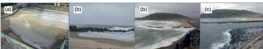
Figure 6. Zurriola beach. (a) Physical Model study (2013). (b) Damage in the 2013-2014 storms and (c) Situation in 2015 after repairs
