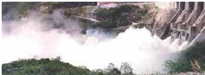
Fig.1 Spray Atomization Phenomena when J Dam Discharging Flood
