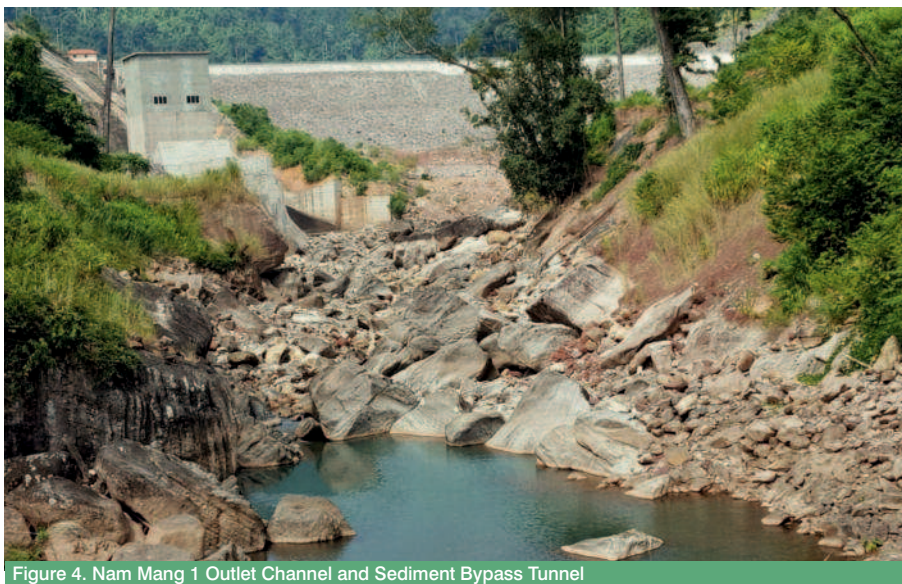
Figure 4. Nam Mang 1 Outlet Channel and Sediment Bypass Tunnel
