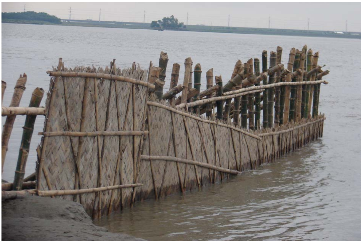
Fig.2. Bamboo fencing attached with the vertical bamboo of Bandalling in the Jamuna River of Bangladesh
