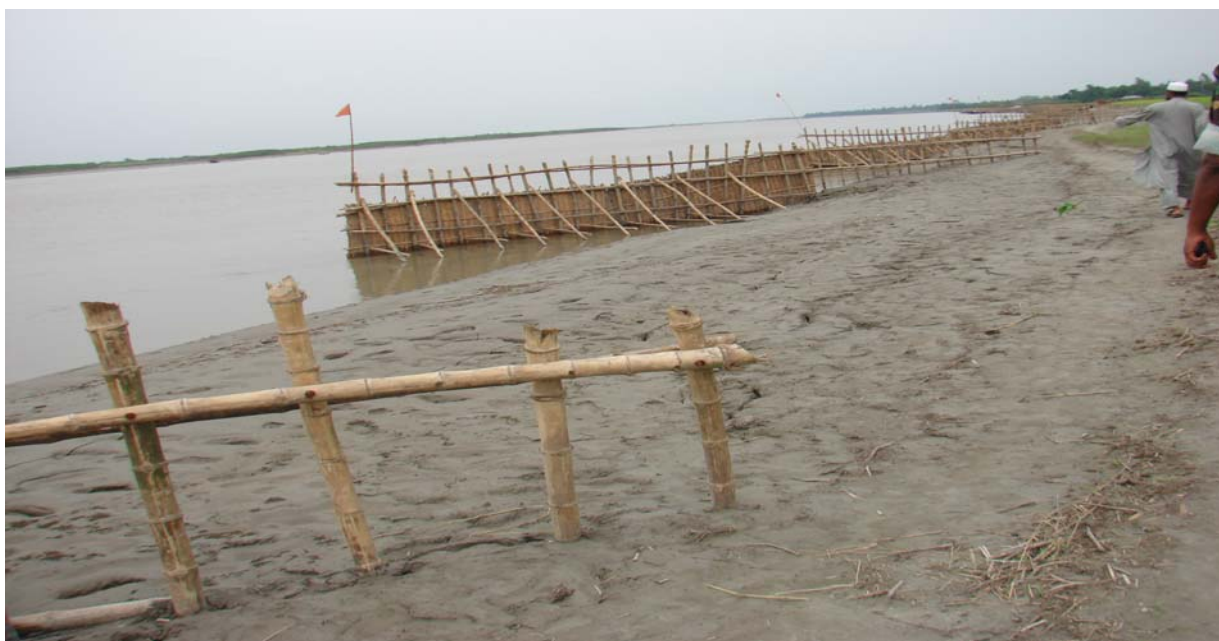
Fig.2. Bamboo fencing attached with the vertical bamboo of Bandalling in the Jamuna River of Bangladesh
