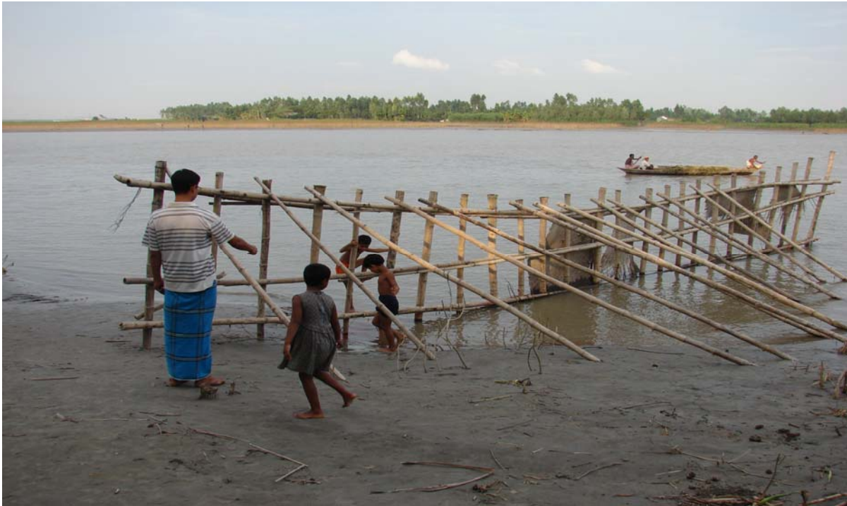
Fig.4. Bandals worked well in the Jamuna River of Bangladesh during the monsoon 2007
