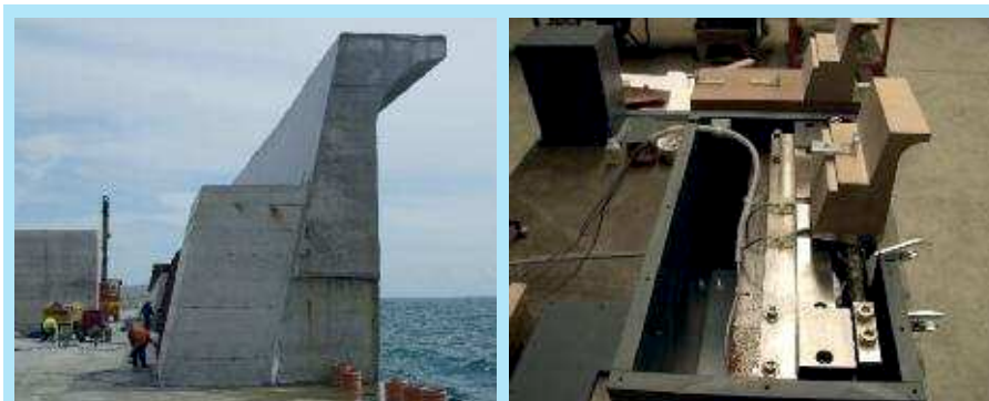
Figure 8. 3-components strain gauge balance for measuring wave loads on the crest wall of the vertical breakwater of Civitavecchia (Italy)
