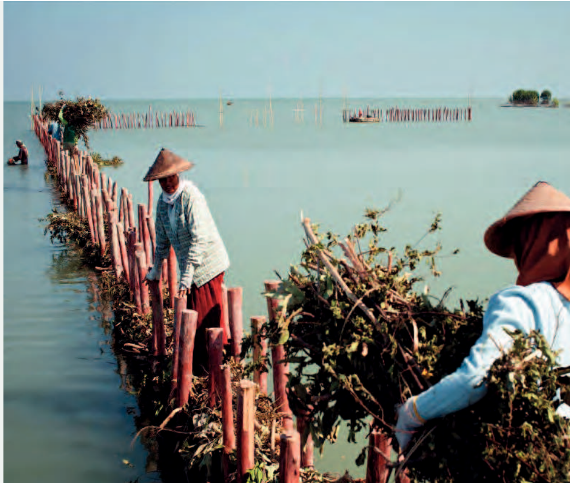
Figure 5 - Restoration of mangrove shorelines in Demak (Java, Indonesia). In March 2015, the Indonesian and Dutch government launched a comprehensive five-year multi million public-private partnership initiative for enhancing coastal safety at the North Coast of Java. It aims to build stable, natural coastlines with reduced erosion risk through a unique integration of mangrove restoration, small scale hard-engineering and sustainable land use. The large-scale pilot project in Demak district focuses on safety against flooding along a 20 km stretch of coastline and sustainable revitalization of 6000 ha of aquaculture ponds. The approach includes a combination of technical and socio-economic measures, as well as creating an enabling environment through stakeholder dialogues and capacity building. The ultimate goal is to enable replication and up-scaling of the concept, for incorporation in a variety of urban and rural development programs.
