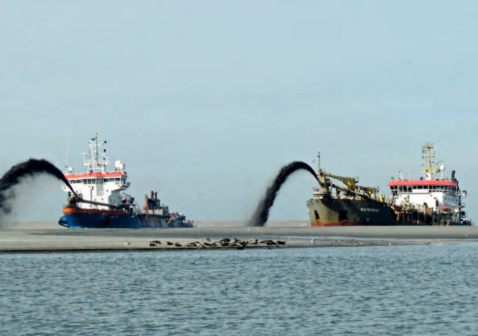
Hoppers of Van Oord (left) and Boskalis (right) working together in the construction of the Rotterdam Port Extension Maasvlakte II.
