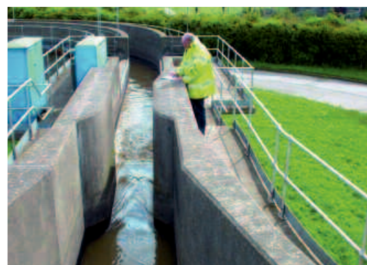
Figure 3 – Inspection of a flume on an effluent discharge channel to ensure compliance with the relevant flow measurement standards
