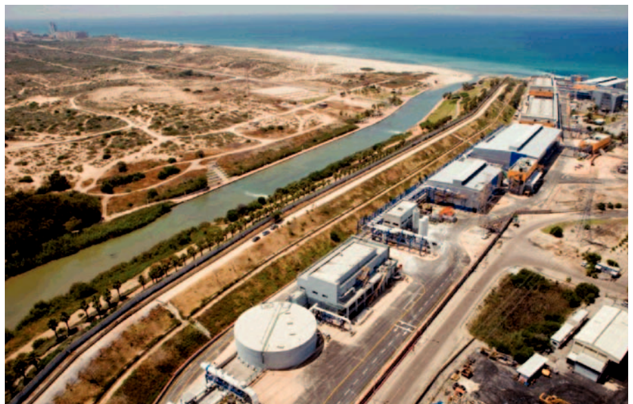
Hadera (Israel), world's largest RO desalination plant (275,000 m 3 /d, source: IDE Technologies)
