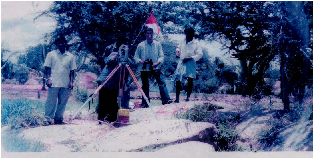
Fig 3 Triangulation survey and fixing the position of range pillars
