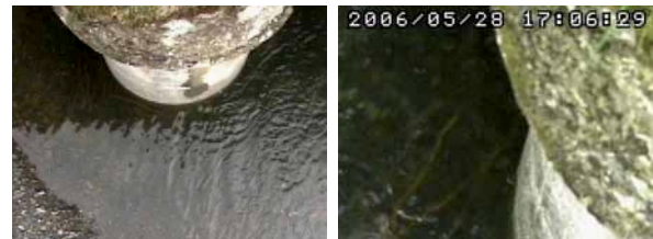
Fig-6 Trees observed around the bridge pier after flood due to snowmelt (right: an image observed at the Sapporo station; left: a close-up of the image)
