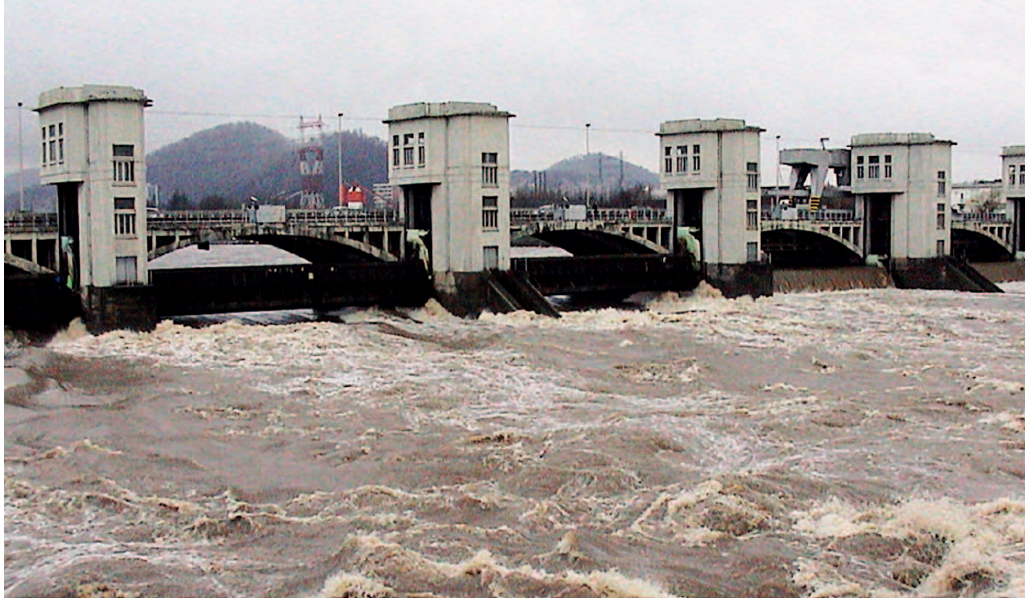
Monsin dam downstream of Liege during floods in February 2002
