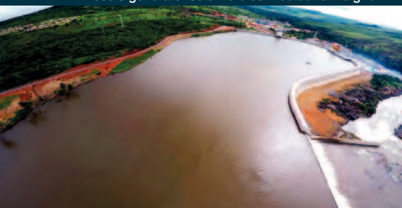
Panoramic view of KALETA Hydropower station, whose 3 generator sets were connected to the grid
