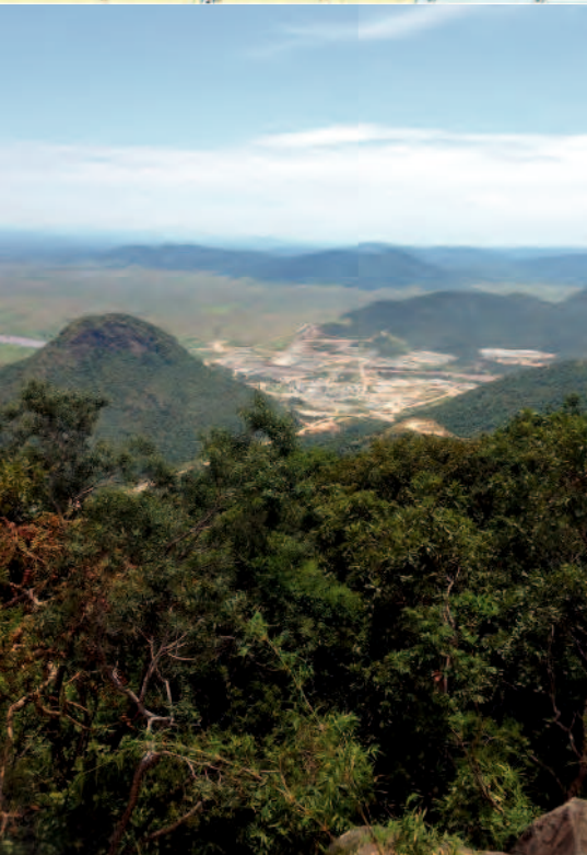
The panoramic view of GERD site from left bank side October 2014
