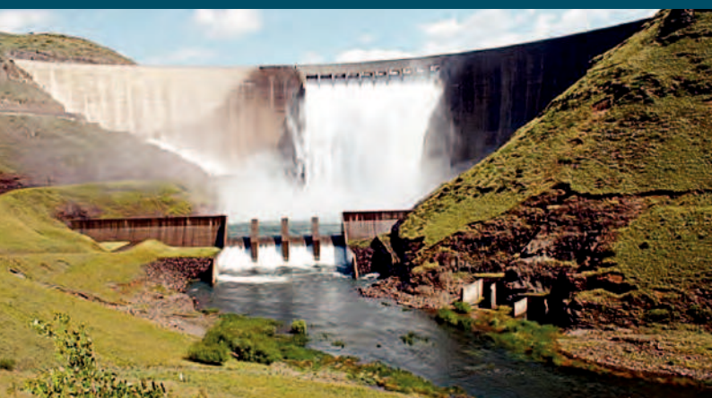
Katse dam in Lesotho at an altitude of 2000 masl.
