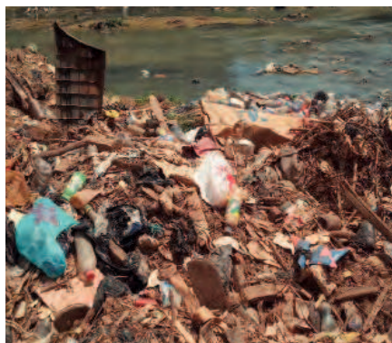
A storm drainage system filled with plastic waste and other debris in one of the cities in Ghana
