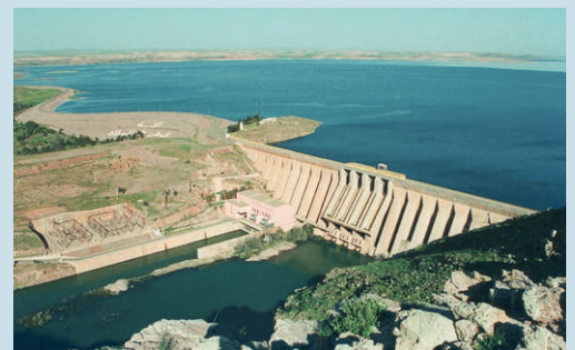
Figure 4. Al Massira dam (service year: 1979, height: 82 m, initial reservoir capacity: 2,785 Mm 3 , sedimentation rate: 2.3 Mm 3 /year), Oum Rbia River, Oum Rbia basin
