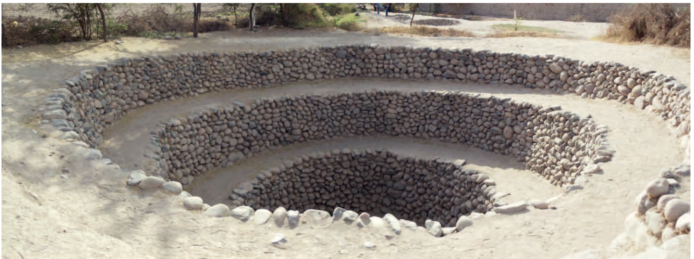
Figure 3. Spiral access hole to filtration galleries in Cantayoc, Nazca. It is located 450 km South of Lima
