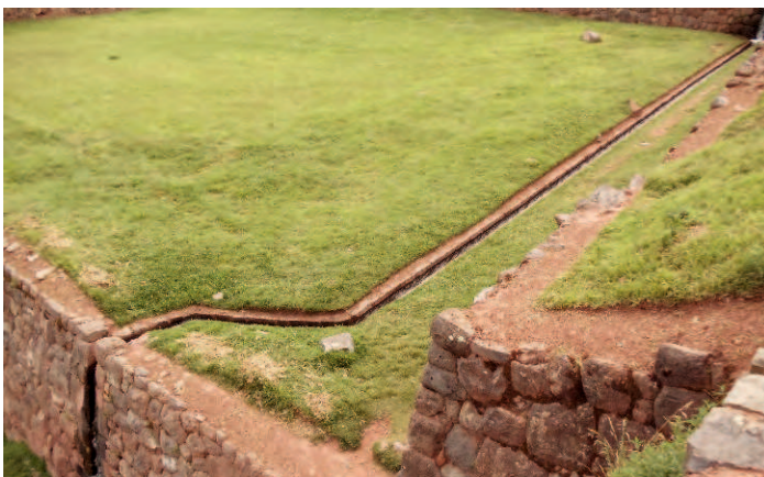
Figure 4. Rock canal and waterfall in Tipon, a small Inca urban center located 24 km South of Cusco City. Notice that energy losses are induced upstream of the waterfall by creating a sinuous path. Consequently, the jet trajectory stays close to the stone wall
