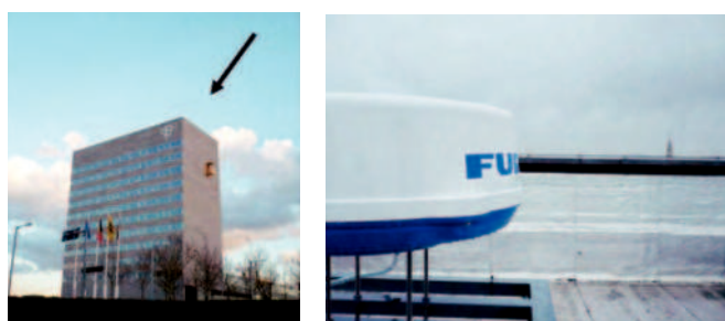
Fig. 2: Location of the Leuven X-band radar of Aquafin, on the roof of the Provinciehuis building.
