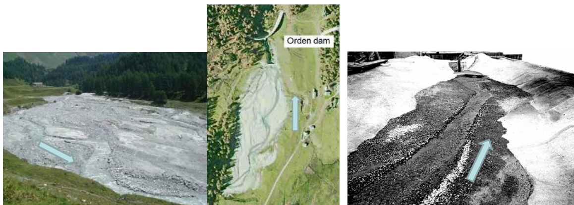
Figure 8 Reservoir sedimentation of Orden dam in Switzerland (Left: From dam to upstream view, Middle: Aerial view, Right: From upstream to dam on the model study)
