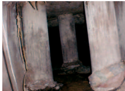
Figure 1. Unplanned obstacles in the collection systems' cross-section in Brazil (source: SUDECAP).
