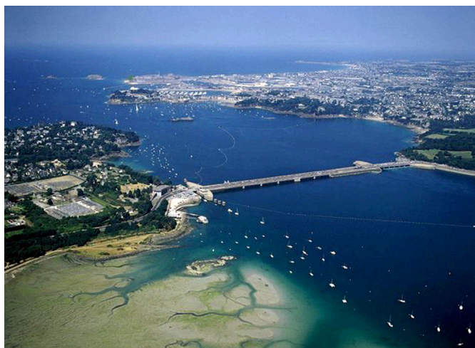
Figure 2 | The Rance Tidal Barrage.
