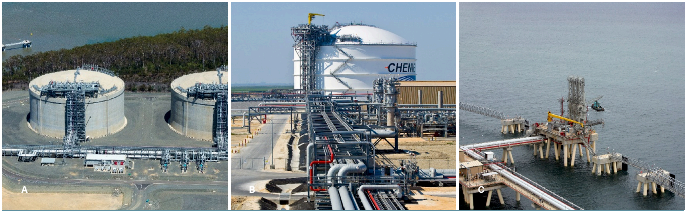
Figure 4 | General view of LNG loading systems. (A) Storage tanks area, (B) Main Loading Lines, (C) Jetty Piping.
