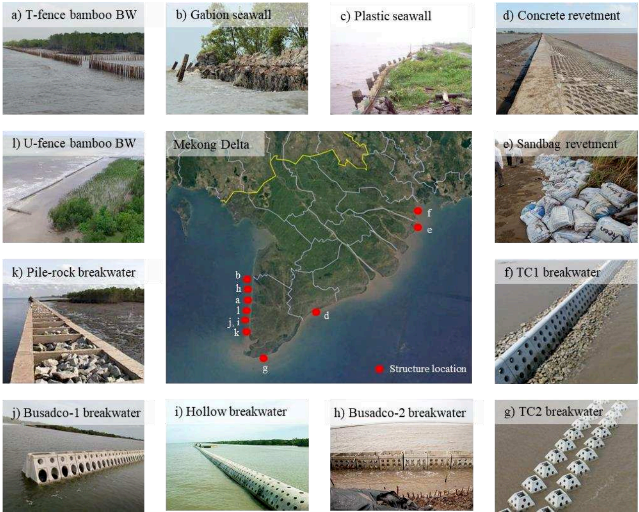
Figure A1: Several existing coastal protection measures in the Mekong Delta (Source: images were collected from GIZ (2016); SIWRR; DARD Camau; and KIT).
