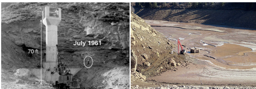
Figure 2. Paonia Reservoir near Hotchkiss, Colorado reached the end of its sediment design life after 50 years when the outlet became clogged with sediment and woody debris. The outlet was constructed in 1961, 21 m above the reservoir bottom (left). By 2014, the sediment level at the dam was 1 m higher than the outlet works (right). Photographs courtesy of Bureau of Reclamation
