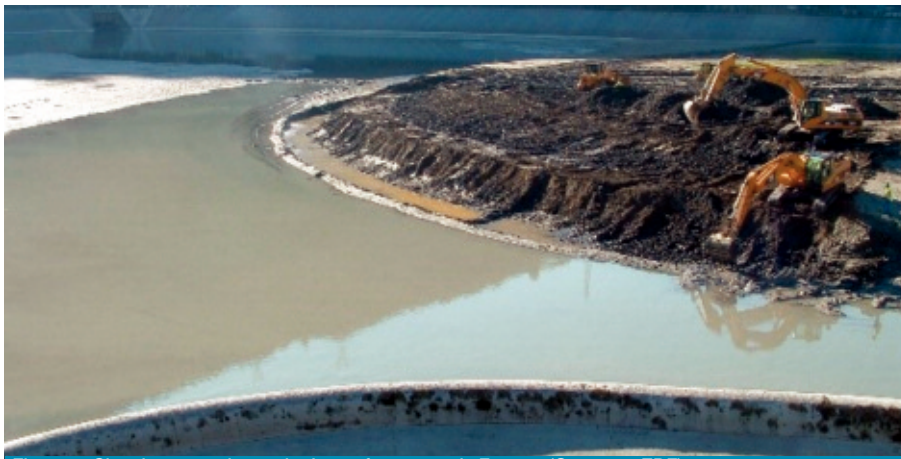
Figure 4. Cleaning operation at the Longefan reservoir, France. (Courtesy: EDF)
