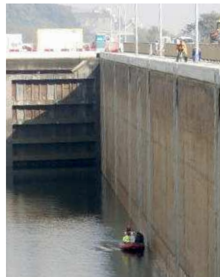
Figure 4. Installing a pressure probe in Lanaye lock chamber
