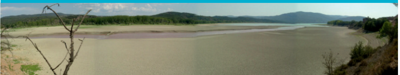
Figure 1. General view from upstream of Barasona Reservoir in Spain. The Barasona Dam was commissioned in 1932 with an initial capacity of 71 Mm 3 , increased up to 92.2 Mm 3 in 1973. Some flushing and dredging operations were conducted in the 1970's and 1990's, and nowadays the live storage capacity of the reservoir is estimated to be around 70 Mm 3
