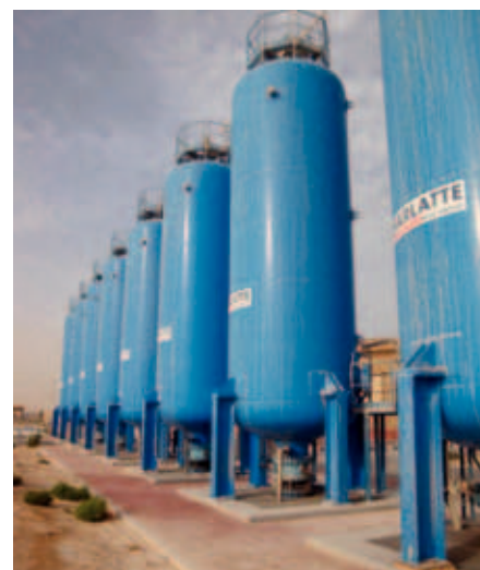
Figure 1. Surge vessels in the United Arab Emirates from [1].
