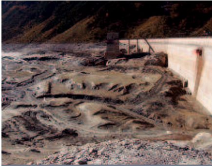
Figure 3. Sedimentation in an Austrian reservoir after a controlled reservoir level drawdown (courtesy: Gökler)
