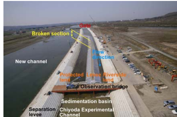
Fig. 1. Levee constructed in the Chiyoda Experimental Channel
