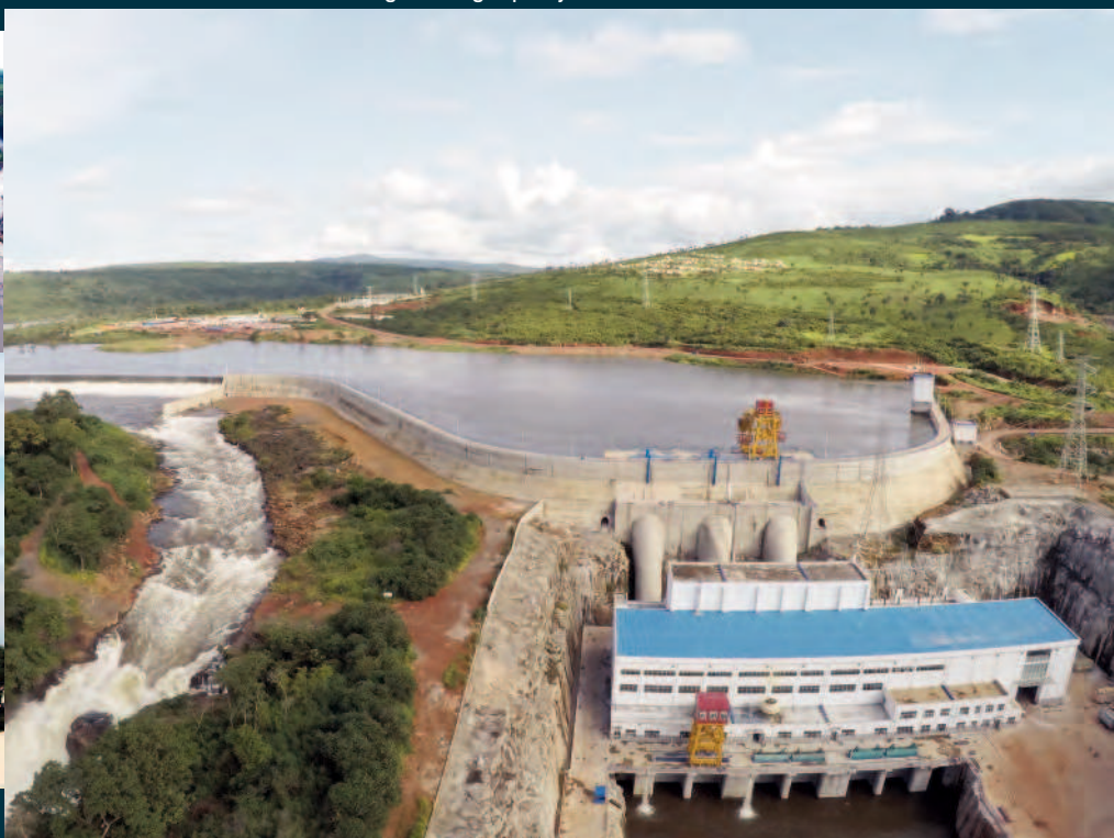
Powerhouse of KALETA, whose annual generating capacity is 965 GWh
