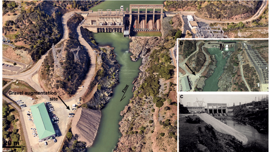
Figure 2. Gravel replenishment below Keswick Dam. To balance the sediment starvation created by trapping in Shasta and Keswick Dams, gravel is deposited from dump trucks down the bank of the Sacramento River, creating a cone to be eroded by subsequent high flows. (a) Remote-sensing composite image of site, showing gravel pile emplaced (15 April 2015), and (b) subsequently eroded (24 May 2017) (Google Earth). (c) Gravel augmentation has been ongoing here for decades, as reflected in a much-reproduced photo from January 1989 by Kondolf.
