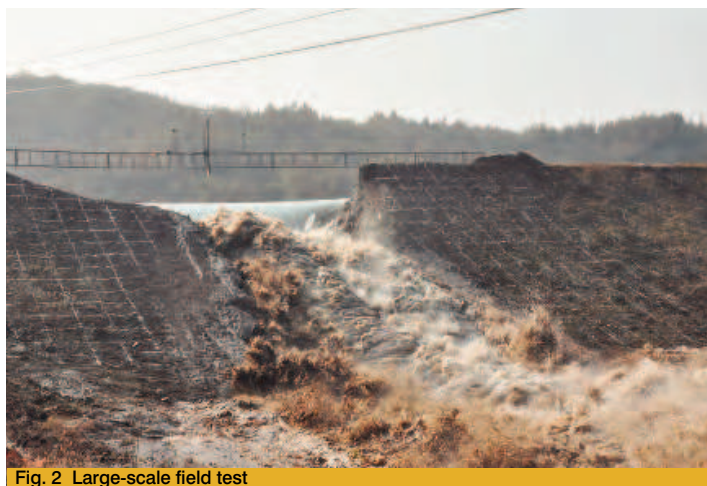
Fig. 2 Large-scale field test
