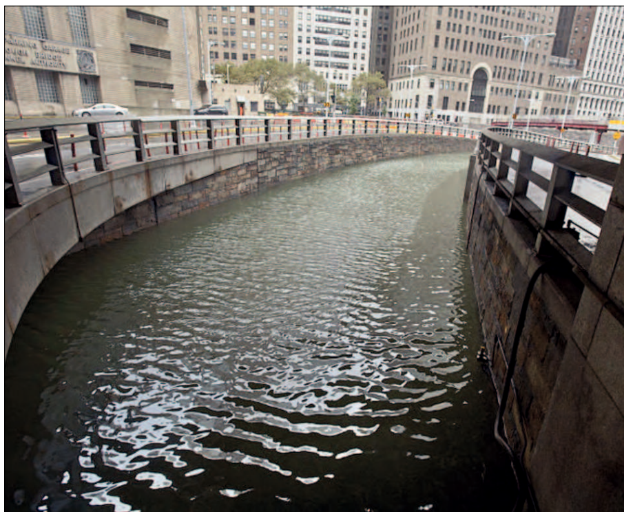
Flooded tunnel in New York City (Photo from Wikipedia).
