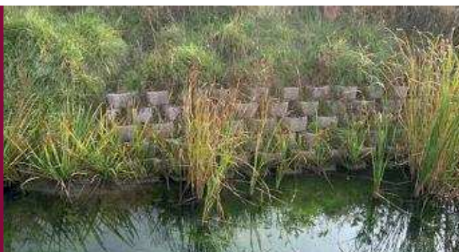
Figure 3. Vegetated block slope protection
