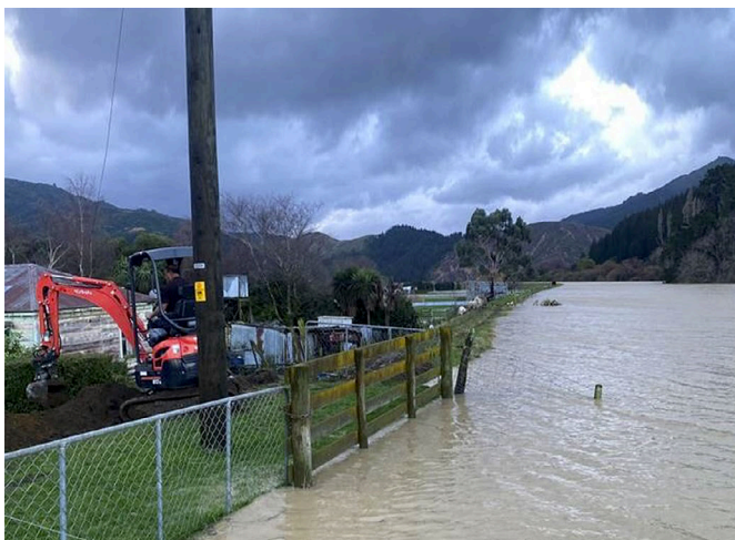
Figure 2 | Flood peak against a key stopbank (dyke) with emergency work to limit overtopping.
