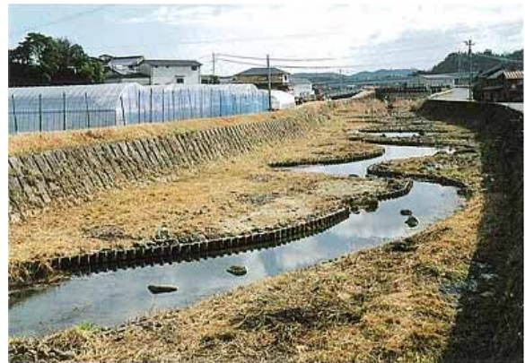
The case of river with fixed channel, although river boundary is wide enough.
